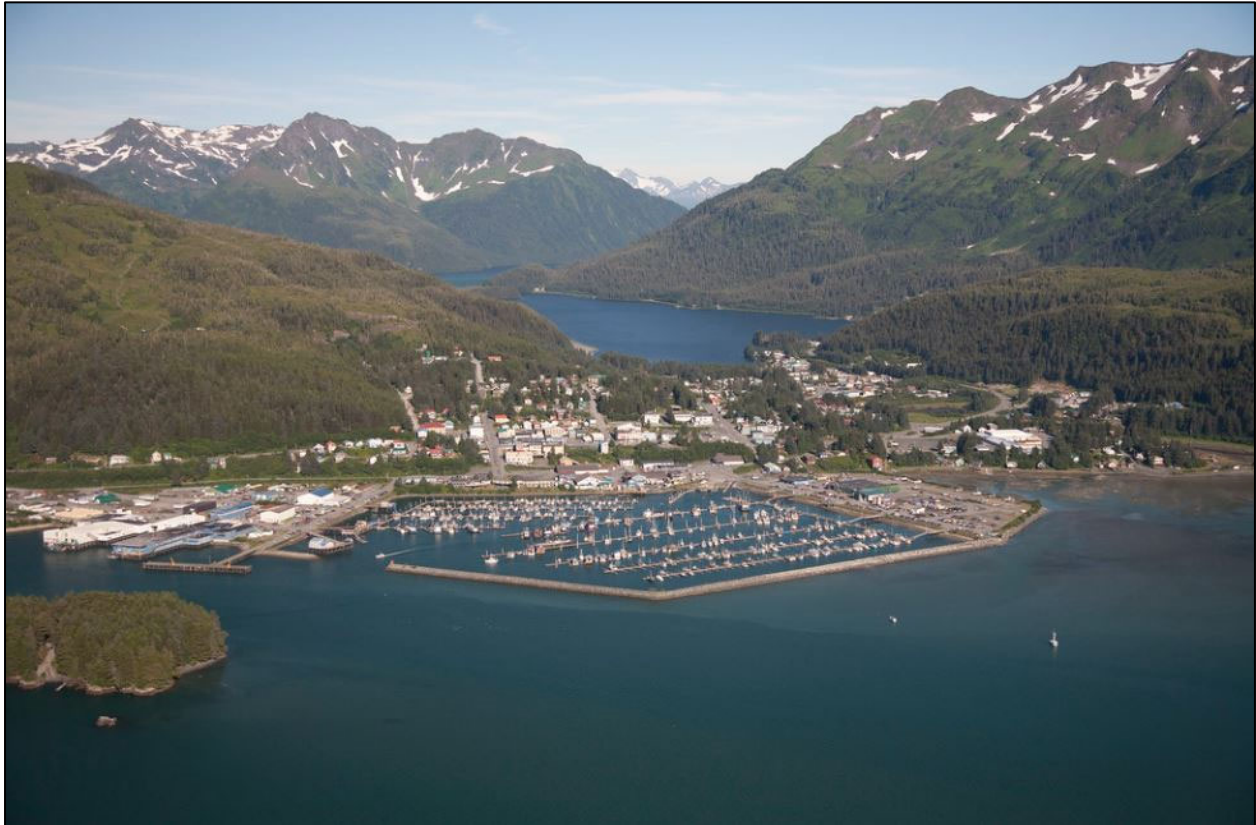
Figure 1. Photo of the Cordova Harbor Rebuild Project Area
